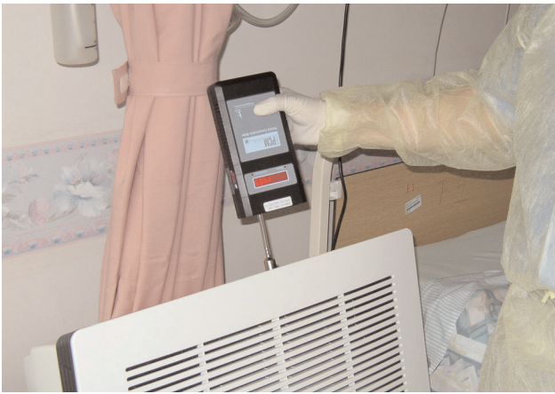
Assessing the actual filtration efficiency of an air cleaner with a laser particle counter.
